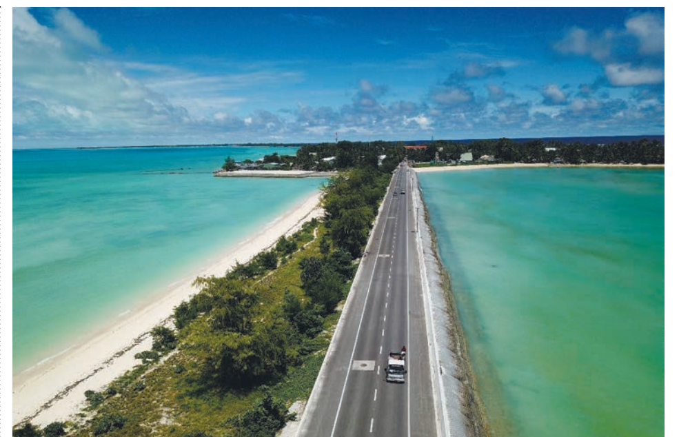
JICA supports economic activities on remote islands such as Kiribati (above) by rebuilding roads damaged by storm surge, a deadly ocean phenomena exacerbated by rising sea levels. JICA
